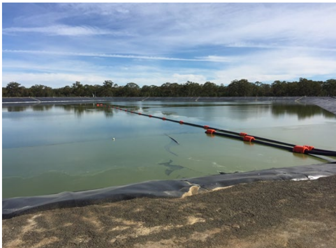
A CSG water holding pond. The reverse osmosis treatment process produces water suitable for uses such as irrigation, livestock watering, or dust suppression, and also produces a reject waste stream which is highly saline (brine).
