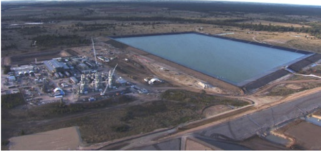
A CSG water holding pond and treatment facility in Queensland.
