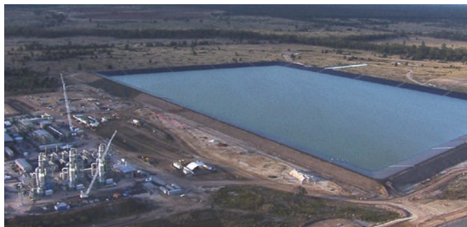
CSG water holding pond and treatment facility in the Surat Basin.
