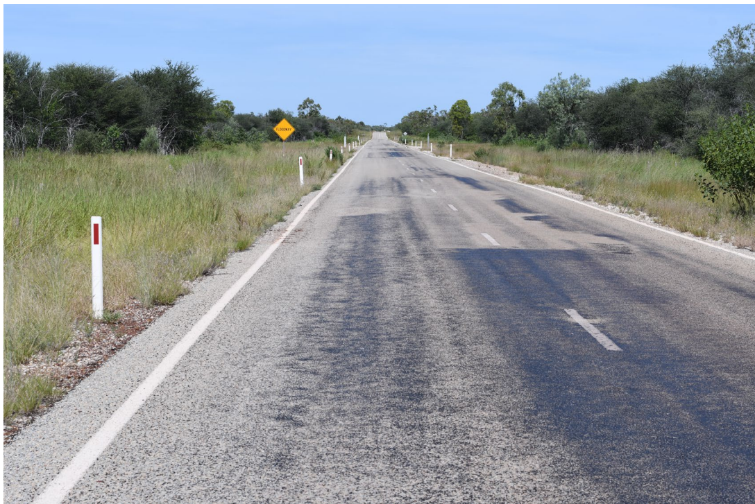
Figure 13 The Carpentaria Highway during the wet season (February 2023) showing the presence of grass up to the edge of the bitumen
