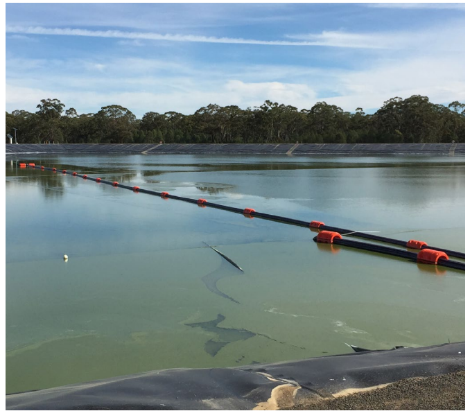
A CSG produced water holding pond.
