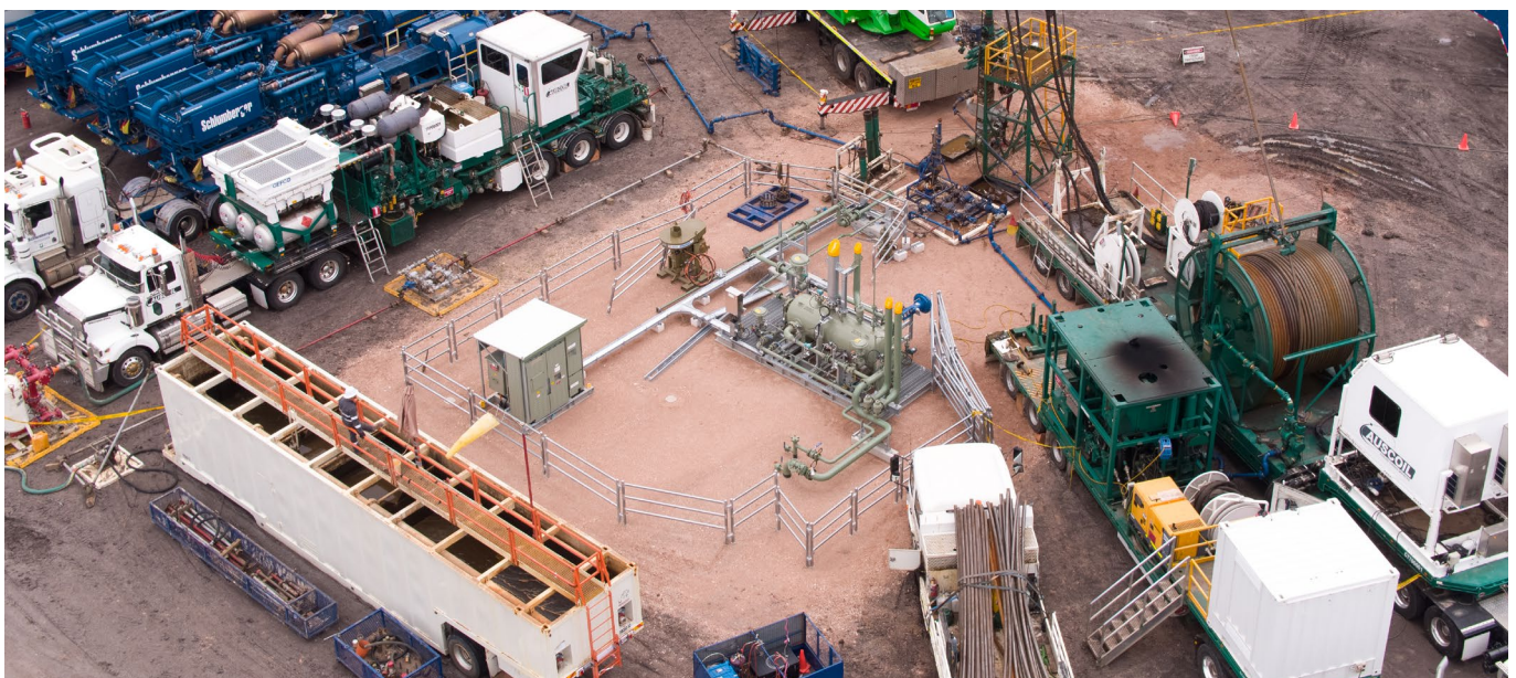
A CSG well site undergoing hydraulic fracturing operations.
