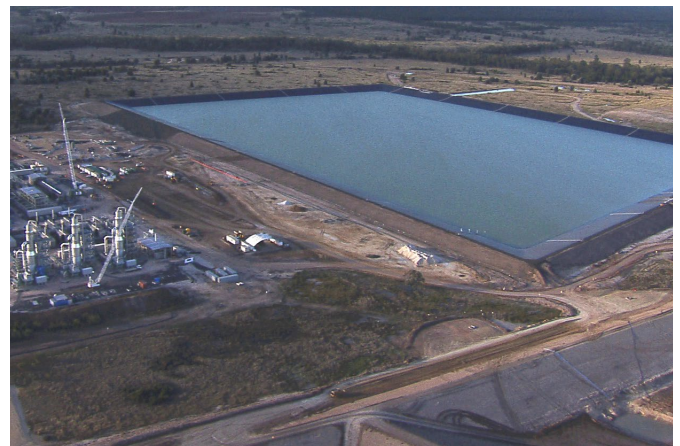
RO plant and holding pond
