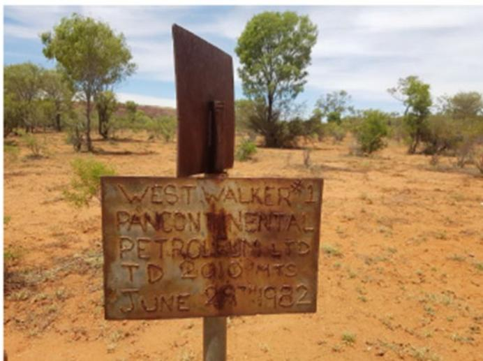
Figure 20: An example of a surface marker for a decommissioned well in the Northern Territory.
