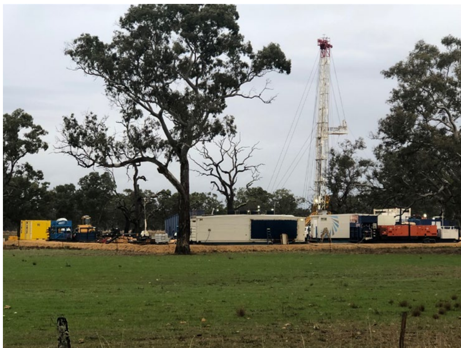
Conventional gas drilling rig
