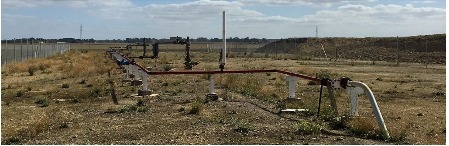
Decommissioned gas well in the Penola region.
