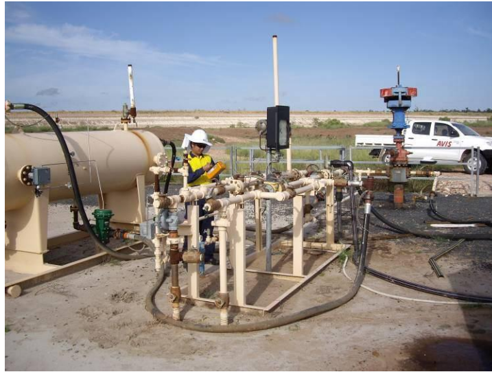
Figure 2: External survey of field well in Talinga region – February 2010.
