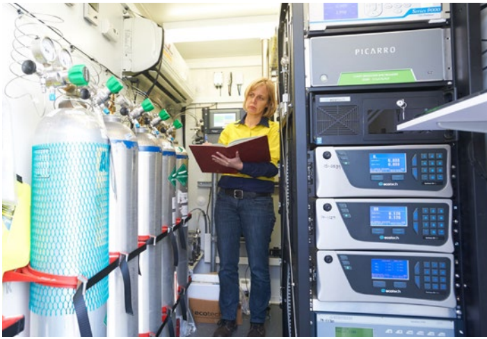
Air monitoring equipment inside the station.
