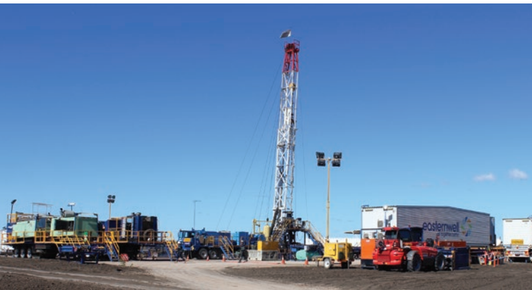
An example of a CSG work-over rig in action on a cultivated field.
